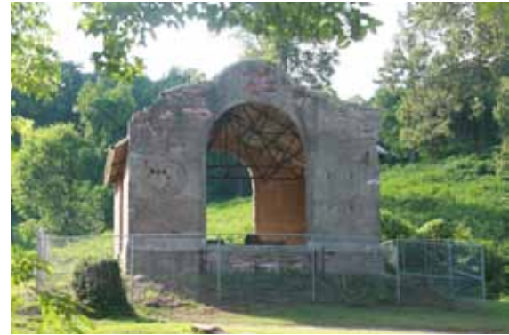
Hoist House - Red Mountain Park
